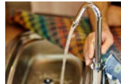
Correct installation of the hydraulic systems.
